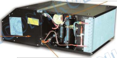
Large evaporator and condenser coils with raised lance fins enhance the system's ability to dissipate heat.
